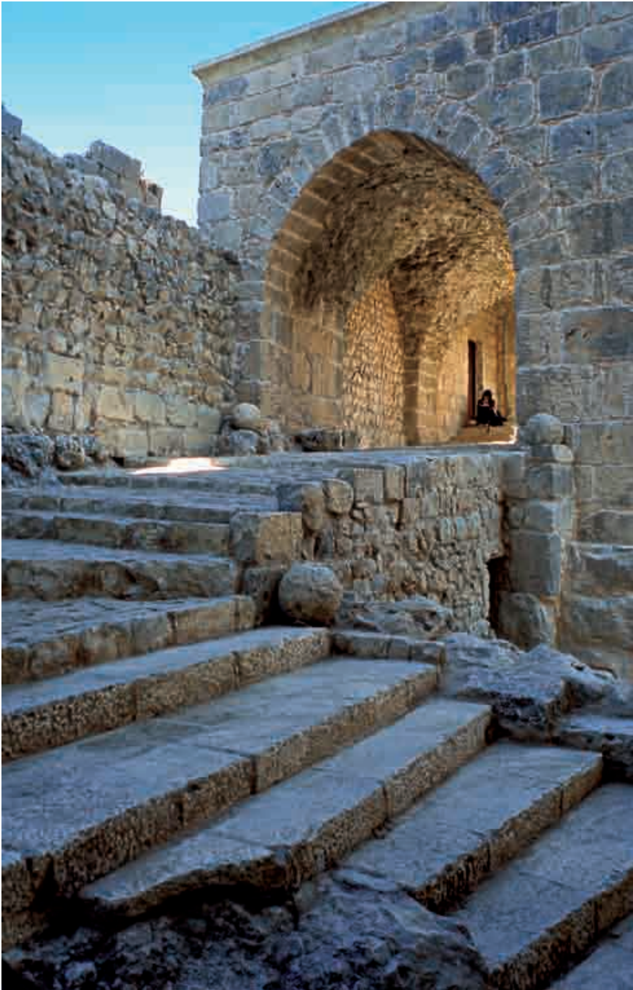
Left, the restored entrance to the upper mosque and madrasa of the Citadel of Salah al-Din.
