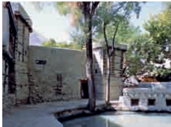
This page, the repaired community pond in Ganish, Pakistan, with restored enclosure walls and towers.
