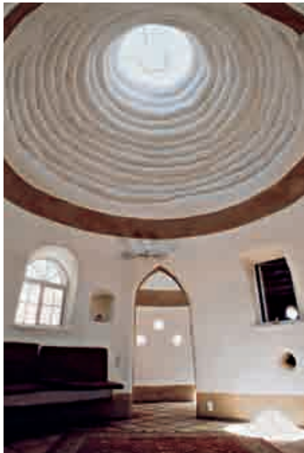
Concentric placement of the sandbags results in this instance in an almost traditional looking architectural environment, with a dome and an overhead oculus.
