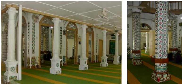
Figure 5: (a) Series of columns located left and right of the mosque's interior; (b) 'Belian' columns with decorative bright colored tiles
