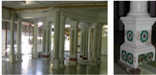
Figure 6: (a) Group of column located at the back verandah supporting the roof structure; (b) Decorative tile located at the base of the column
