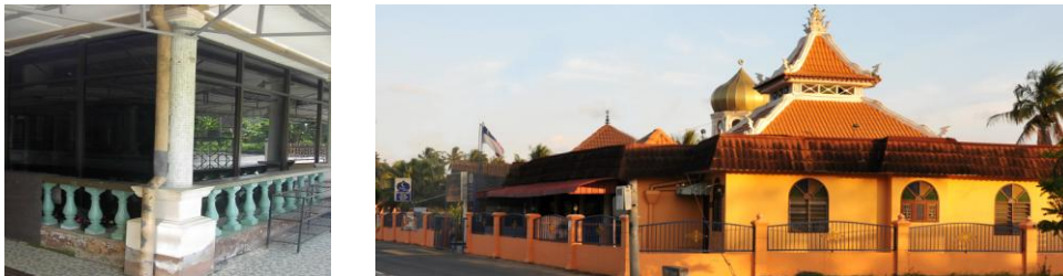
Figure 3: (a) Glass door addition to overcome the street noise problem; (b) Kg Rim mosque recent photo looking from Jasin-Nyalas main road (source: e-masjid/portal Masjid Negeri Melaka portal)
