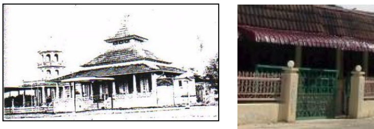
Figure 10: (a) Old photo showing the original front porch main entrance; (b) Recent photo showing metal gate installed after the glass door at main entrance
