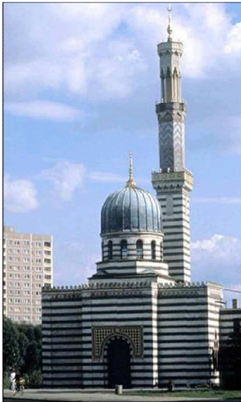
Fig. 3 Steam Driven Pump Station, Potsdam, Germany, Ludwig Persius, ca. 1842
