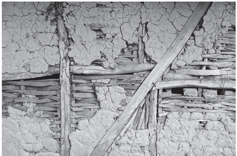
Figure 14. Wattle-and-daub remains in the vicinity of the Atik Mosque (Photo by E. Jahić)
