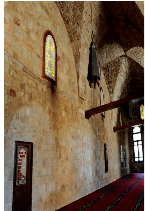
Figure 85: Colored glass fenestration located at the Qibla wall to avoid glare.
