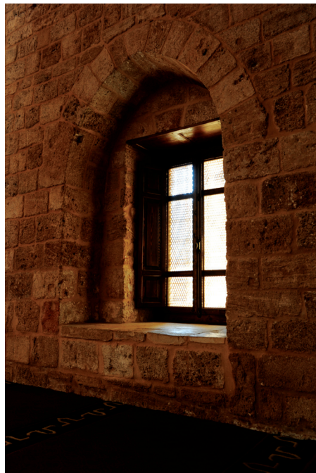
Figure 86: Small recessed windows, located at the western part of the prayer hall, allowing daylight to enter the space in the afternoon.
