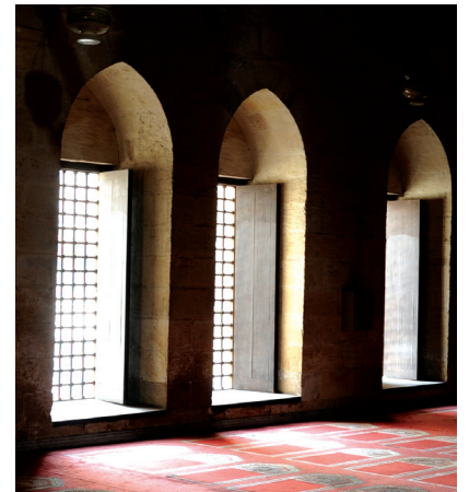
Figure 36: 970 Al-Azhar Mosque vertical recessed windows reduce the amount of contrast between interior and exterior spaces.
