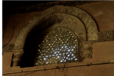
Figure 64: All four walls of the mosque are pierced by over 120 pointed arched windows containing delicate filigree grilles, allowing diffused light enter the prayerhall.
