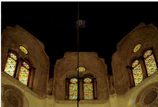
Figure 37: 1295 Sultan Ibn Qala'un Complex Color ed glass windows reduces the strength of sunlight through color filtration mostly used as a decorative element.
