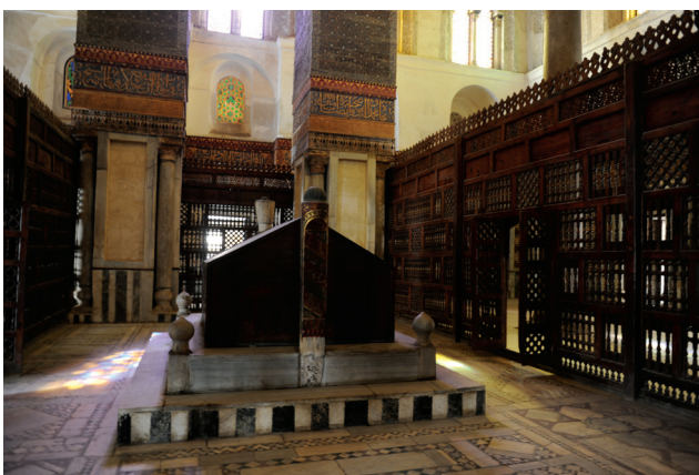
Figure 38: 1295 Sultan Ibn Qala'un Complex Mashrabiya's main function is to scatter sunlight in order to reduce its strength.
