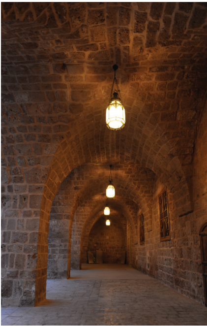
Figure 101: Repeated row of centralized small single source lamps are placed in the Riwaq.
