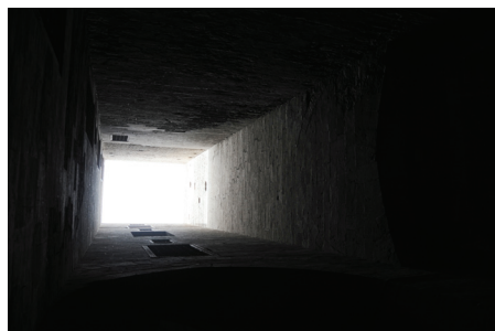
Figure 107: Light shaft allowing daylight to enter the corridors.
