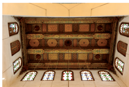
Figure 54: Mihrab windows: bigger windows are located above the mihrab area in order to allow daylight to enter the space from the higher ceiling where the mihrab area is located.
