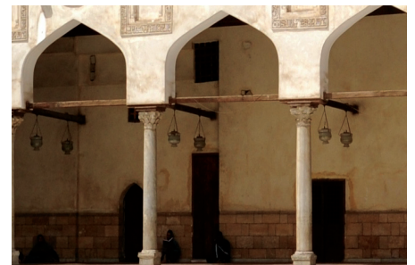
Figure 80: Exterior view of the Riwaq, with hanging mosque lamps.
