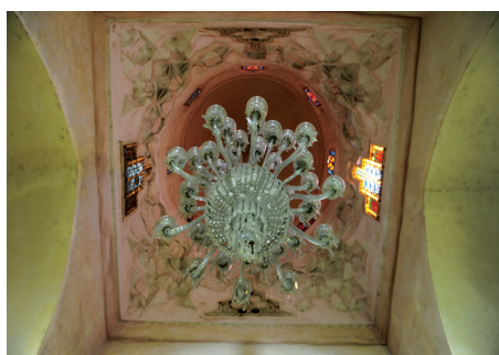
Figure 74: Muqarnas dome with colored glass fenestration, located on top of the Mihrab area.
