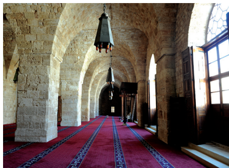
Figure 84: Vertical clear glass windows at the northern part of the prayer hall, where most of the daylight is entering the space.
