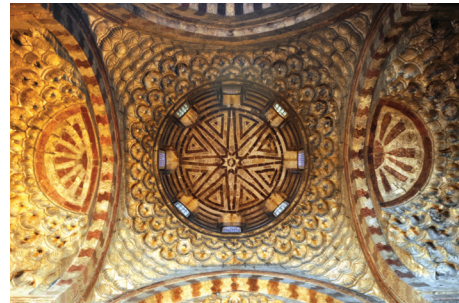
Figure 106: View of the dome located at the main entrance hall, allowing daylight to enter the space through its windows.
