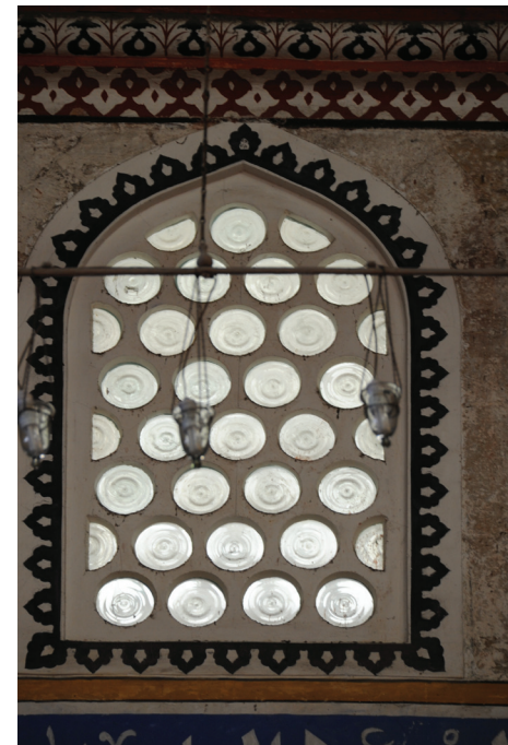
Figure 120: Close up view of the diffusing glass window where most of the day light is allowed to enter the space.
