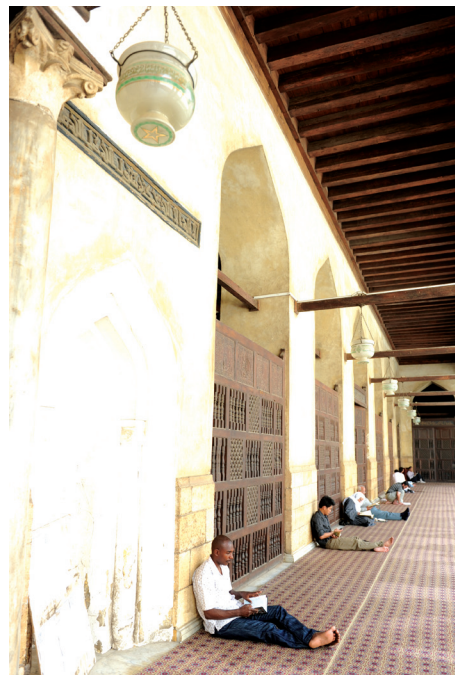
Figure 73: Masrabiya located at the opening of the prayer hall arcades next to the courtyard.
