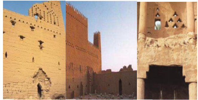
Fig. 2: The details lancets and ventilation triangles of Subalat Mudi in Dir'yyah. Source: (Facey, 1997, p. 104, p. 95). [8]
