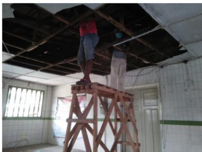
**Figure 5.** Ceiling renovation prior to the demolition (source: Heri Tirtayasa)
