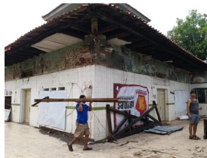
**Figure 6.** After demolition of the intrusive porches (source: Heri Tirtayasa)
