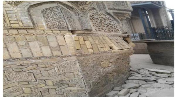
**Figure 3.** Failures in masonry decoration of tilting side of minaret
