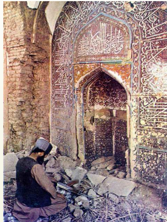
Figure 7. The main prayer hall after the roof destruction in 1985 (photo by Sikorsky; translated by Ahrary 1989).
