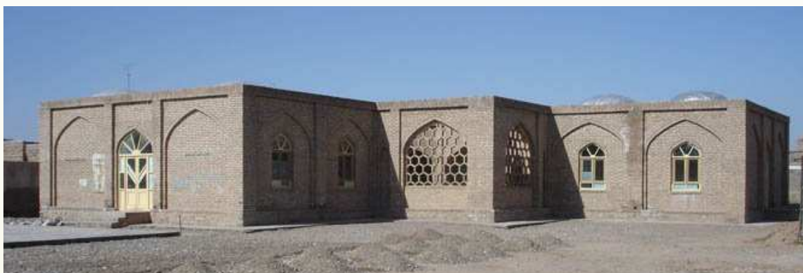
Figure 21. South-eastern view of the school building (2005).
