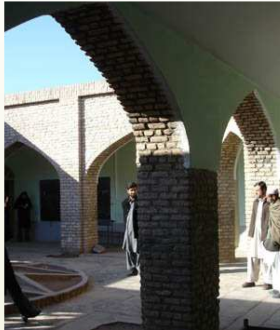
Figure 22. The protected patio linking the two corridors building (photo 2005).
