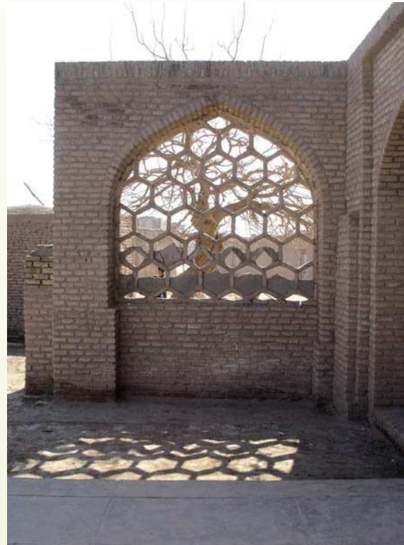
Figure 14. Screen of brick work implemented in the mosque and school buildings.
