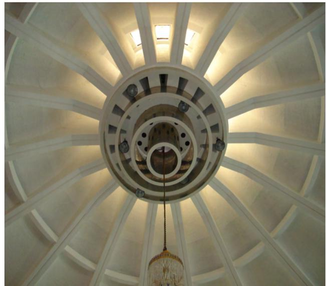
Figure 5.66 Concrete ribbed roof structure with metal ring (Ismail 2007)
