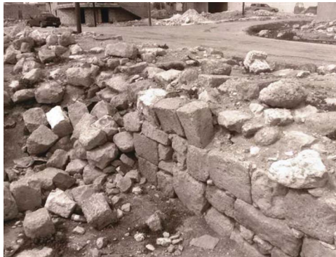
Figure 11. Photograph of the base of Arc Stone (Qantara), which holds the roof in Hayan Mishref Mosque (color figure available online).
