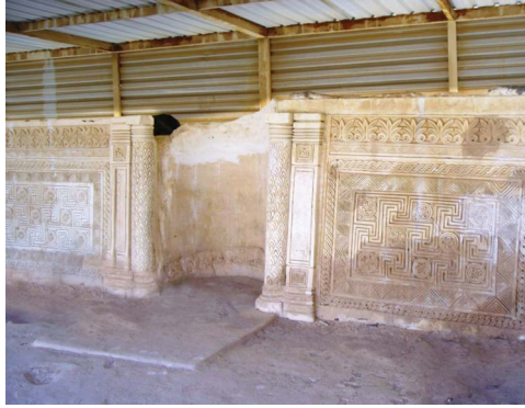
Figure 7. Photograph of the Qibla and Mehrab wall in the Fudayn Mosque showing the stucco decorations after restoration (color figure available online).
