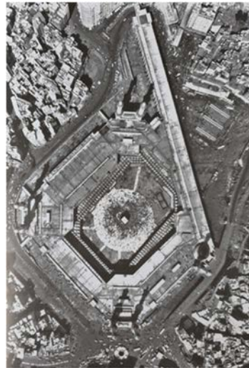
Figure 13: The Holy Mosque after completing the connection with old structure in 1975. (Source: Mirza, 2016, p. 254.)
