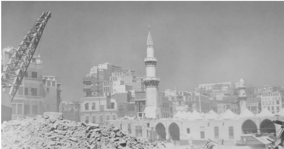
Figure 5: Demolition on the south side of Holy Mosque. (Source: Mirza, 2016, p. 234.)
