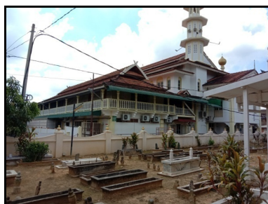
Figure 8. The front view of the Old Mosque Langgar, Kota Bharu, Kelantan was built in 1874 (Image by: Wahid & Abdullah, 2019)
