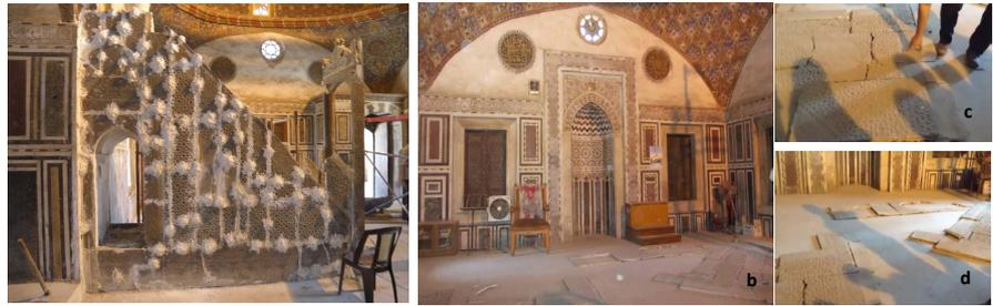
**Figure 3.** The minbar through the reconstruction processes by technicians of archaeological workshops unity of archaeology ministry in 2104. (a) the patches of gypsum mortar for fixing slabs and the inner construction; (b) the aggressive staining of marble slabs of minbar and how amount of dusts and uncontrolled environmental conditions as shown in (c), (d).
