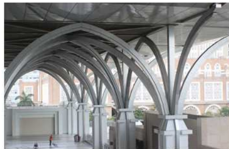
Fig. 6: Masjid Mizan : A language based on 'structural armature' and focusing on the logic of structural forces as in the arch.
