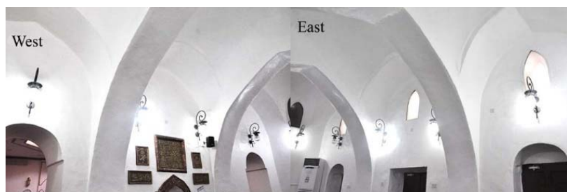
Figure 10: The northern and southern arches are perpendicular to the Qibla wall. They are based on the Qibla wall and the eastern wall opposite it. They also show the roof of the Mosque with the smaller vertical beams on it. (Source: From the work of the researcher.)
