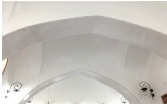
Figure 11: Shows the elongated dome, the roof of the Mosque and its base on the two vertical arches on the Qibla wall, and two the small arches parallel that of the Qibla wall. (Source: From the work of the researcher.)
