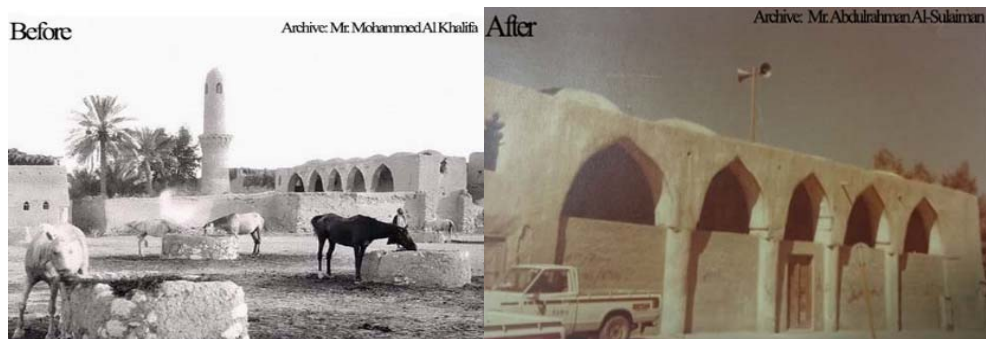
Figure 5: Al-Fatih Mosque in Al-Kut District before and after the demolition of the minaret. (Source: Kalifa and Sulaiman, 2016.)
