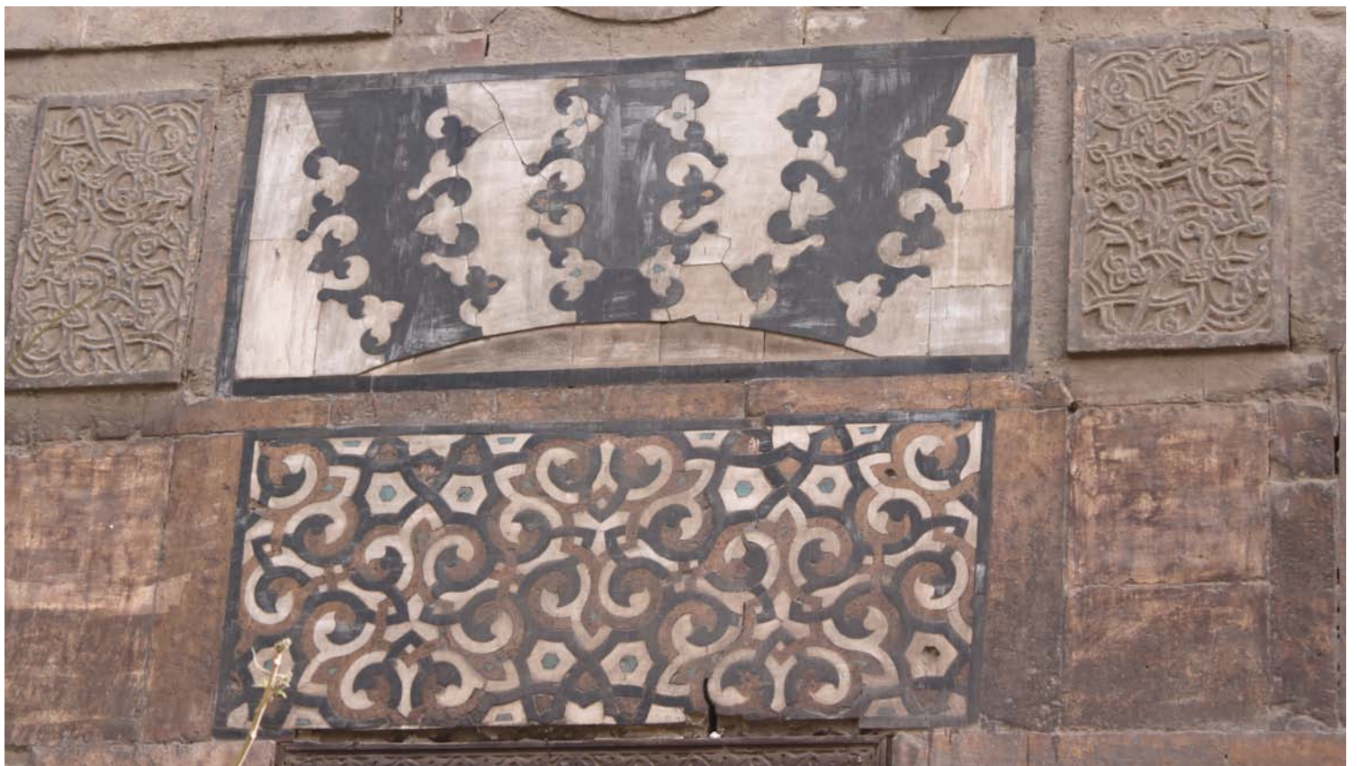
Fig. 4.36: Inlaid marble panels on the northwest façade
