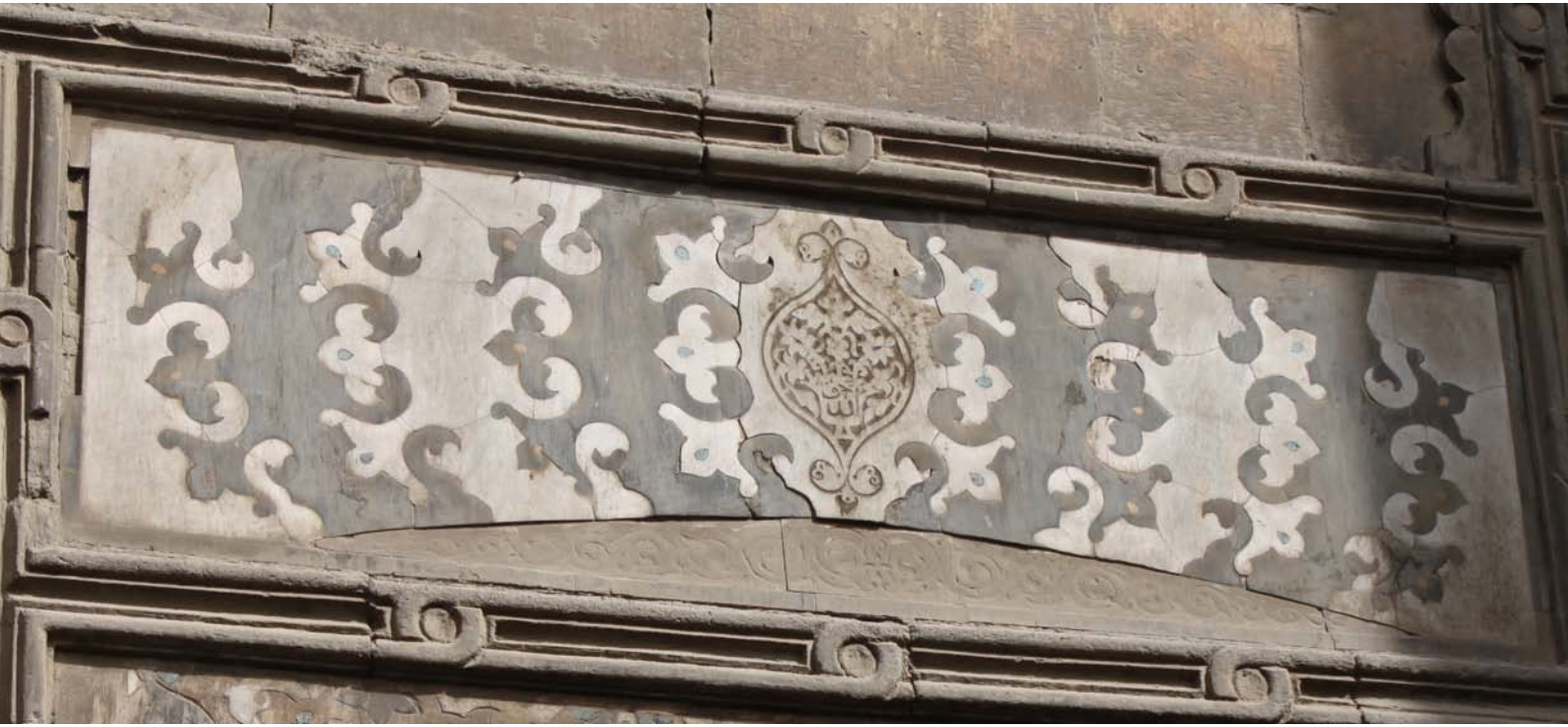
Fig. 4.37: Trefoil panel on the sabil façade
