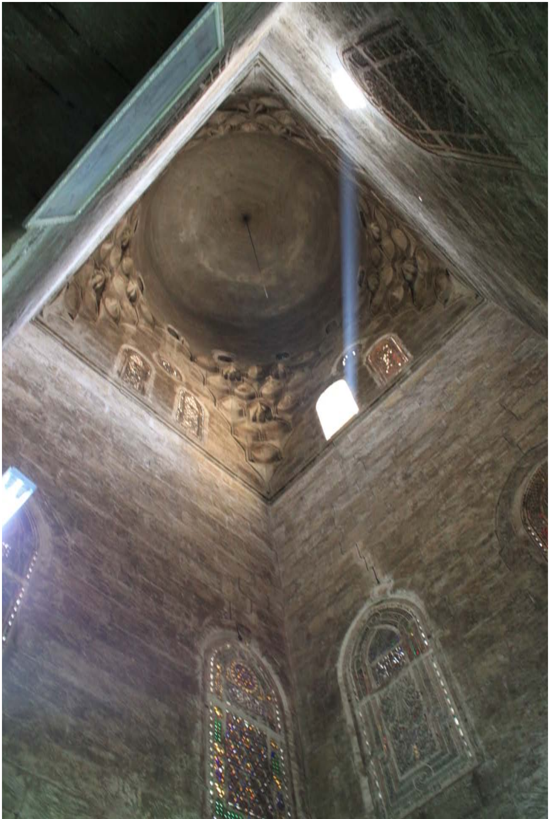
Fig. 4.29: The mausoleum dome viewed from the interior
