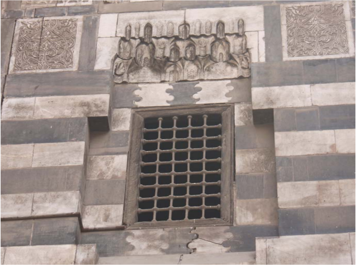
Fig. 4.13: Window with muqarnas hood in the mosque of Qijmas al-Ishaqi
