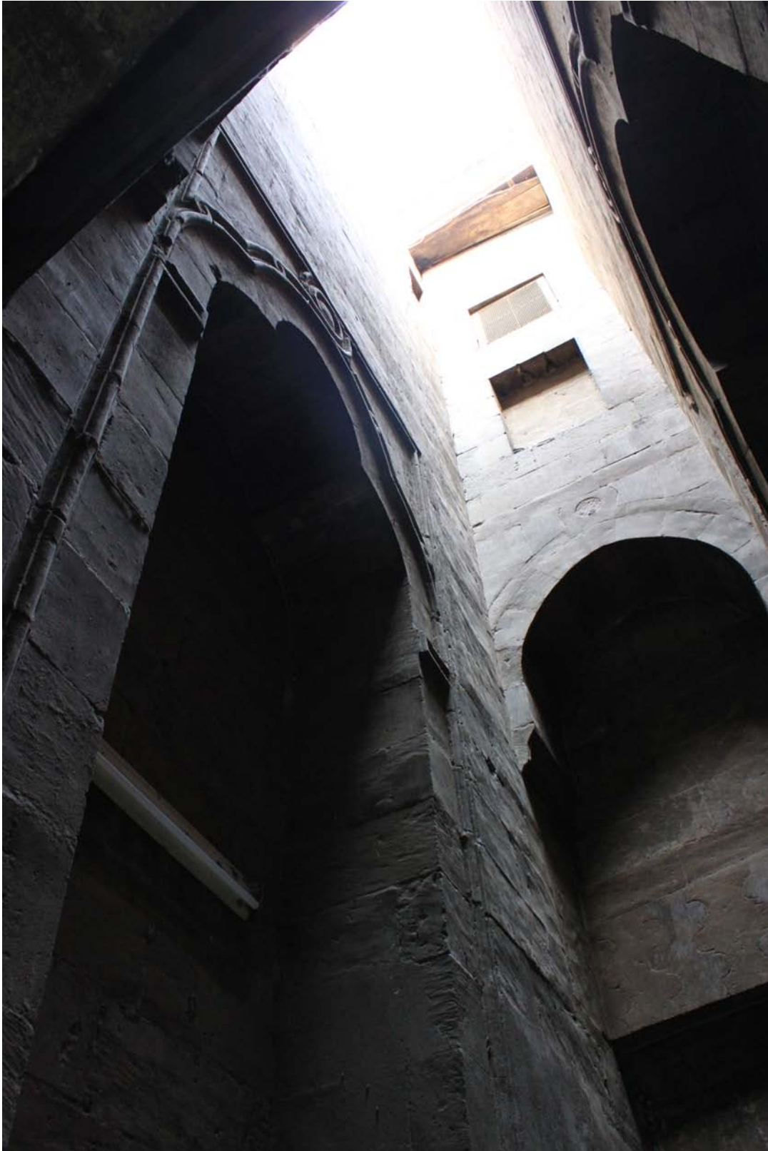
Fig. 3.11: The open-air passageway leading from the entrance vestibule into the sahn
