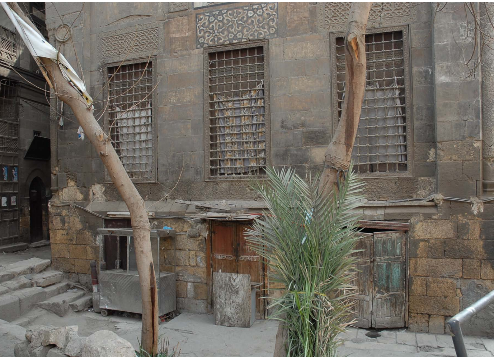
Fig. 2.5: The shops at street level on the northwest facade
