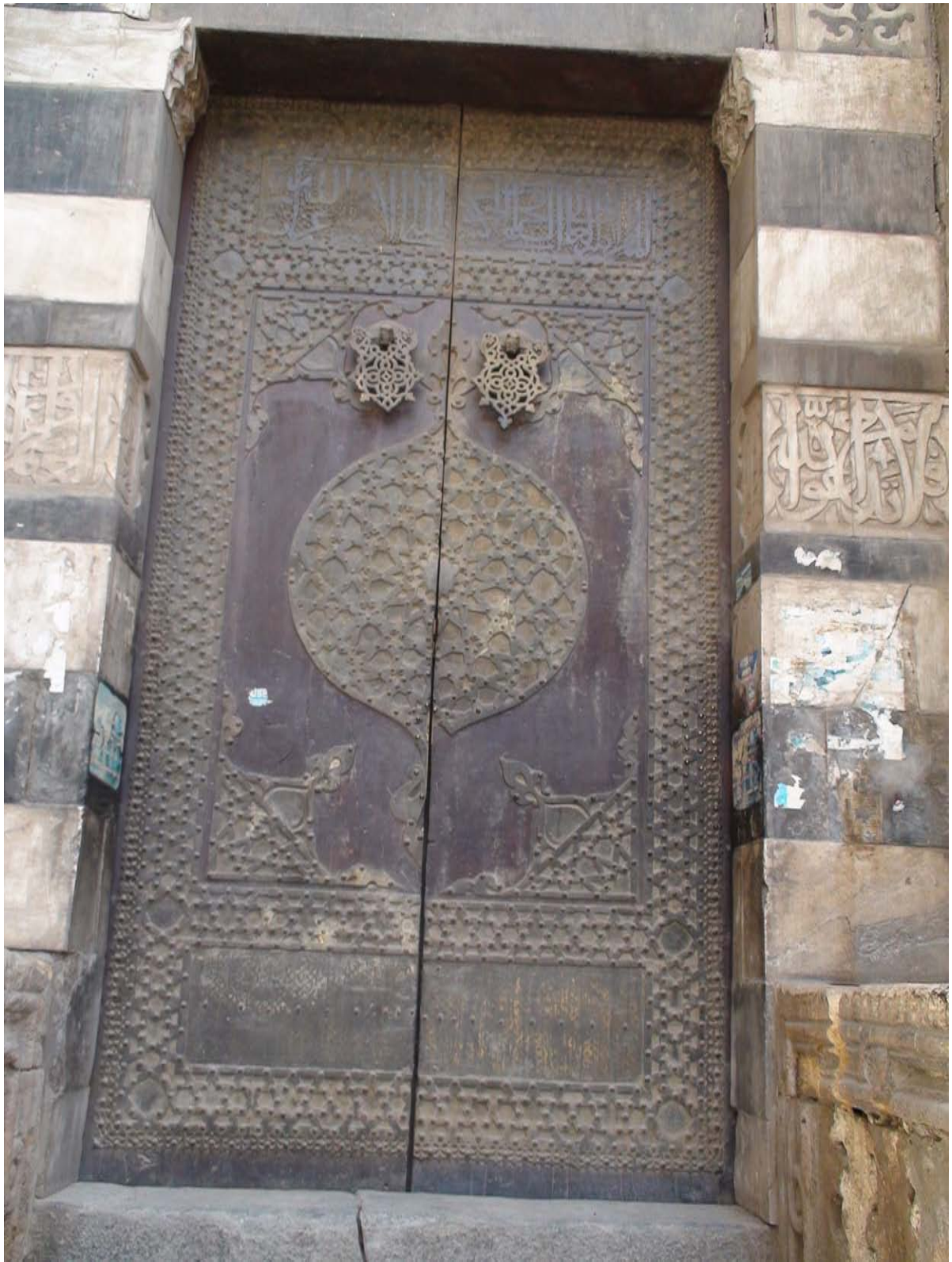
Fig. 4.19: The metal revetted door of the main portal
