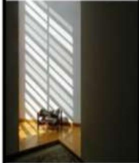
Corner edges are left unmet to create a corner lightwell by wall washing with adjacent opening.
