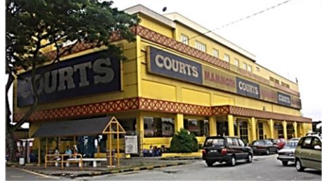
4 Storey Shopping Complex at Jalan Genting Klang, Setapak, for Rohas Sdn Bhd
