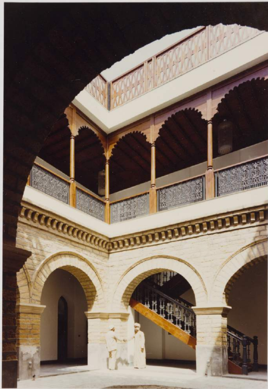
Courtyard Details of Restoration of Traditional House, Muscat.
