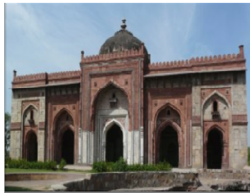
Fig.14. Mosque at Old Fort
