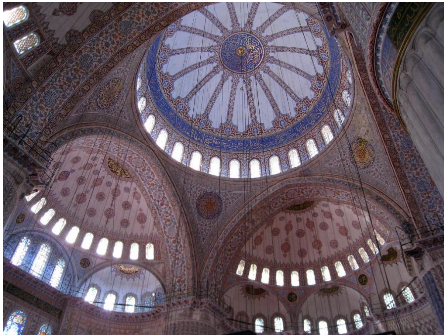
Figure 38. The windows around the main and semi domes in Sultan Ahmet mosque (Blue mosque), (by author in 2012)
