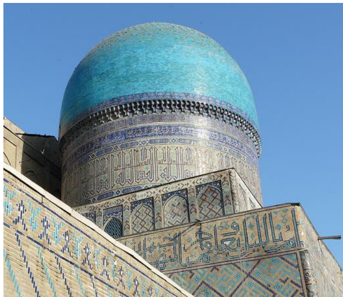
Figure 54. The main dome of the Bibi-Khanym Mosque, (Sele, 2016)
