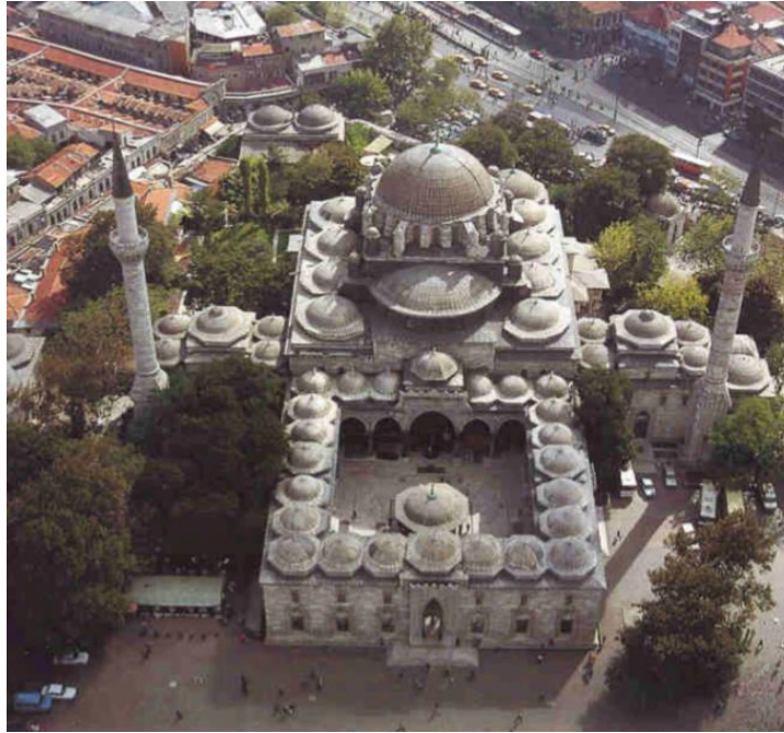
Figure 33. Bayazid II Mosque, all domes are getting a rise toward center dome, rising and bed-chamber, or interior prayer hall is joining to courtyard, (Hattstein M. D., 2000)
