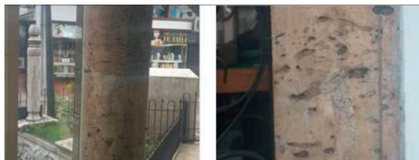
FIGURE 5: Degradation of stone on masonry piers.
