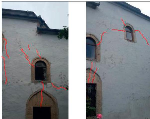
FIGURE 4: Crack inspection at load-bearing walls.
