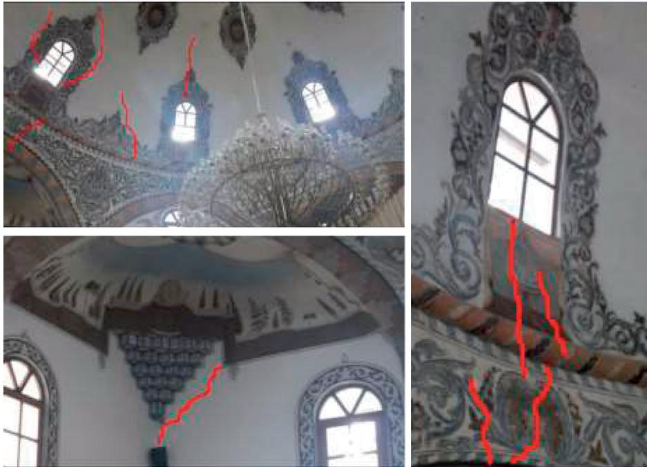
FIGURE 3: Crack inspection at domes, arches, and pendentives.
