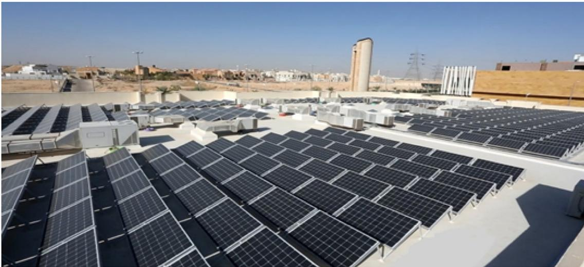
**Fig. 7.** The installed and commissioned solar PV system on the mosque's rooftop.
