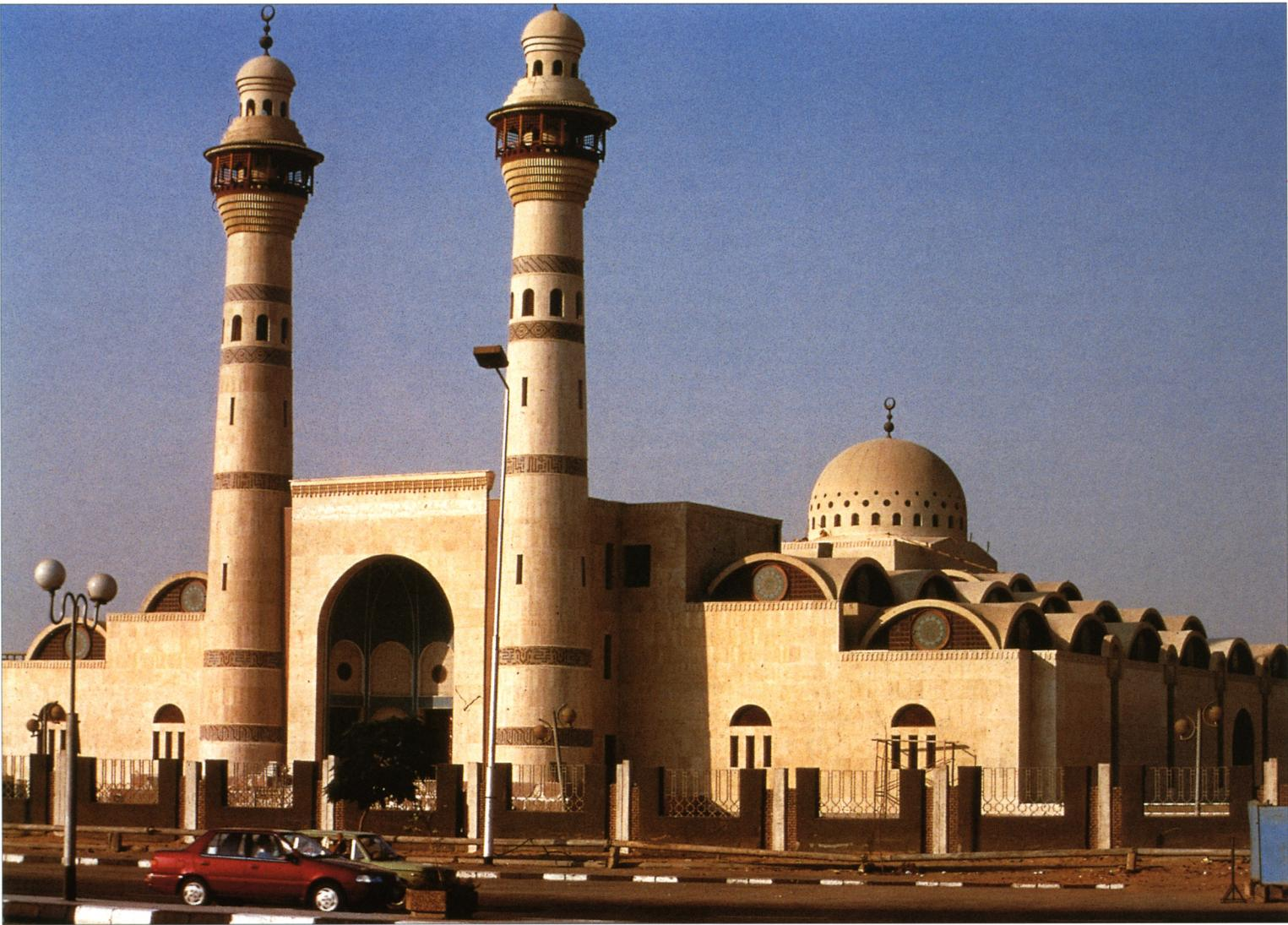
span, thereby avoiding columns in the classrooms. A dome, 8 metres in diameter and 20 metres high, covers the centre of the *qibla riwaq*. The two circular minarets rise to 23 metres, flanking the entrance whose gateway is shaped as an oversized *mihrab*.
