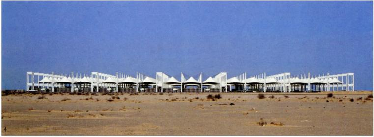
struction of the tent unit is unusual. Unlike most tents its lowest edge does not touch the ground but is some six stories, or 20 meters, above it, with the fabric rising to 33 meters. The fabric surface is supported by thirty-two steel radial cables, which span from the upper tension ring to a lower tie-down or catenary. The twenty-one tent units of each module were raised simultaneously into place by means of electronically synchronized equipment.
