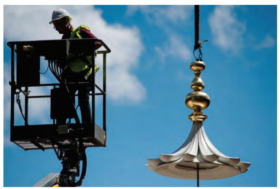
Fig. 207 - New dome finial being placed
